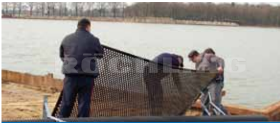
Perforated sheets made of Polystone® G black for the separation of pond zones Placas perforadas de Polystone® G negro para separar zonas en estanques
