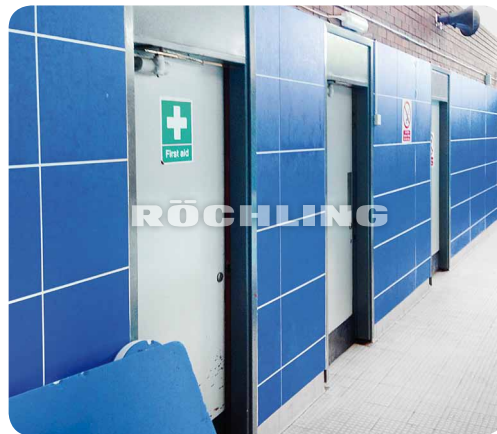
Wall cladding to pool
