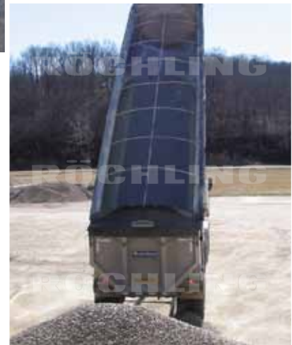
Professional lining: Z-sheets attached to the truck bed prevent material from drifting under the lining sheet
