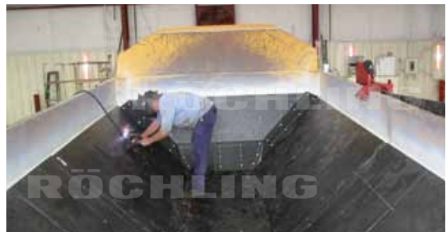
Strongly anchored: Installation of Matrox® sheets in a funnel-shaped dump truck using the stud-welding process
