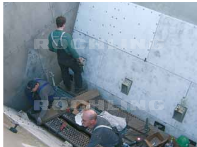
Stud-welding process: lining a hopper
