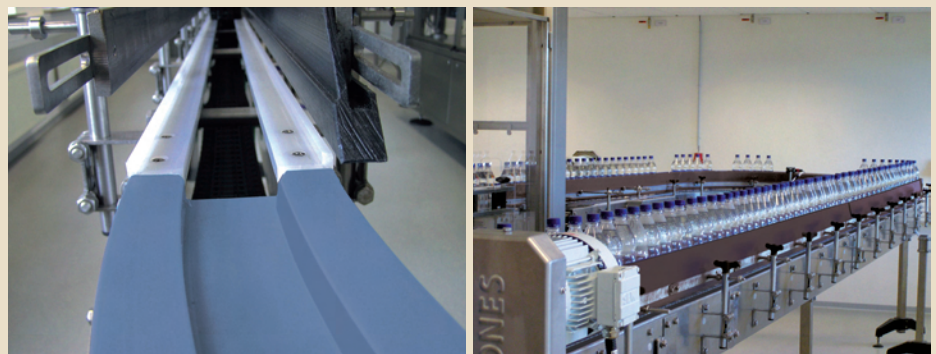
Fig. 2 Bottle conveying plant in the test field in Haren
